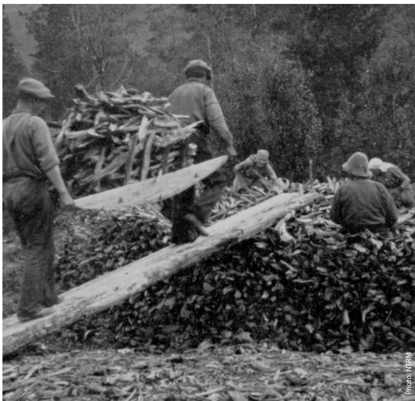
Building a tar kiln in the 1930s - a task that required many hands, and the entire family would often contribute.
